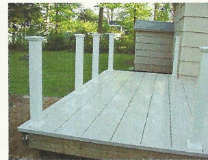
Sleeve PVC Posts over post mounts, measure bays, fabricate & install.
