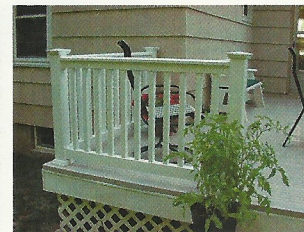
Sleeve PVC Posts over post mounts, measure bays, fabricate & install.
