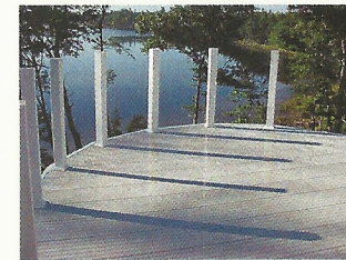
Sleeve PVC Posts over post mounts, measure bays, fabricate & install.
